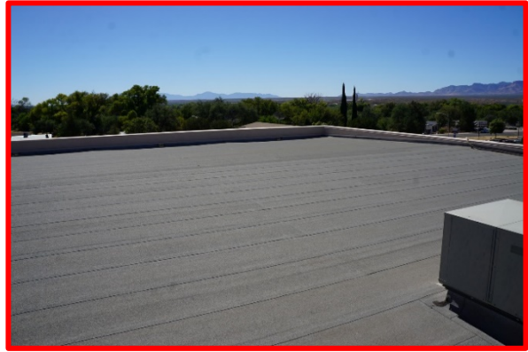
Overview of upper elevation low-slope Bituminous roof system.
