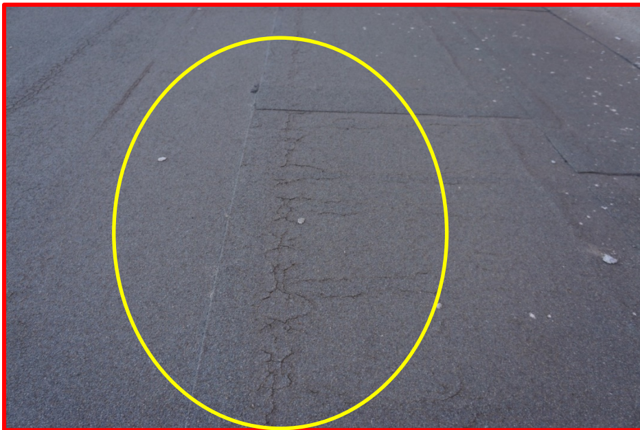
Lower roof cap sheet is alligatoring 1 and cracking, most likely due to UV exposure.
