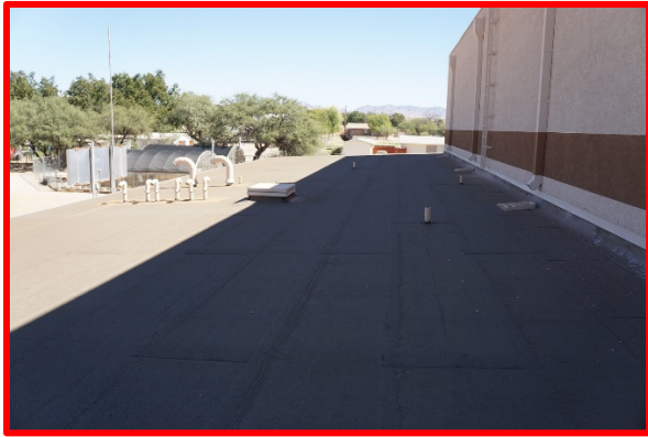
Overview of lower elevation low-slope bituminous roof system.
